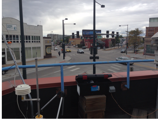
(a) The Denver air quality monitoring station.
